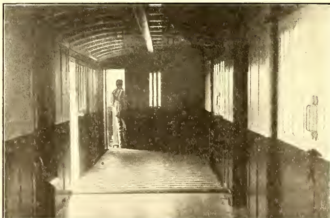
INTERIOR VIEW OF NEW INTERNATIONAL RAILWAY EXPRESS CAR
